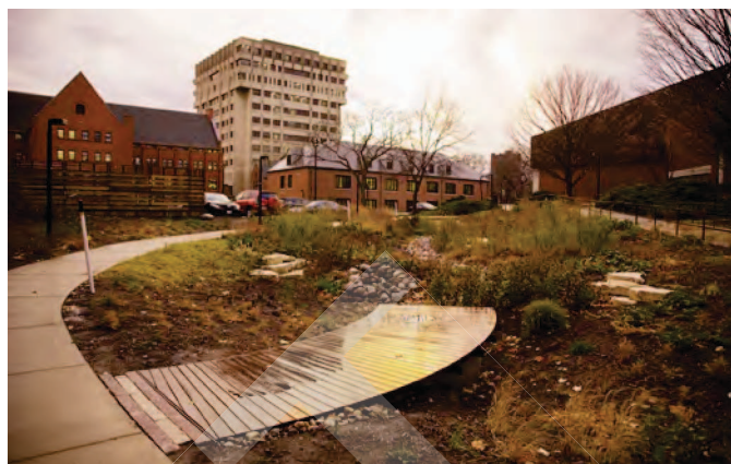
EXAMPLE OF A STORMWATER TREATMENT TRAIN
