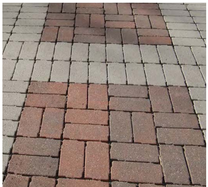
PERMEABLE PAVING - UNDERNEATH THESE PAVERS IS A POROUS SYSTEM OF SOIL AND GRAVEL READY TO FILTER WATER AND SLOW IT BEFORE IT REACHES RIVERS OR STREAMS.
