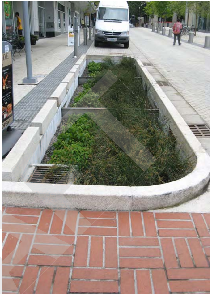
YET ANOTHER EXAMPLE OF A VEGETATED INFILTRATION SYSTEM, MEANING A SYSTEM THAT ALLOWS WATER TO SOAK THROUGH IT.
