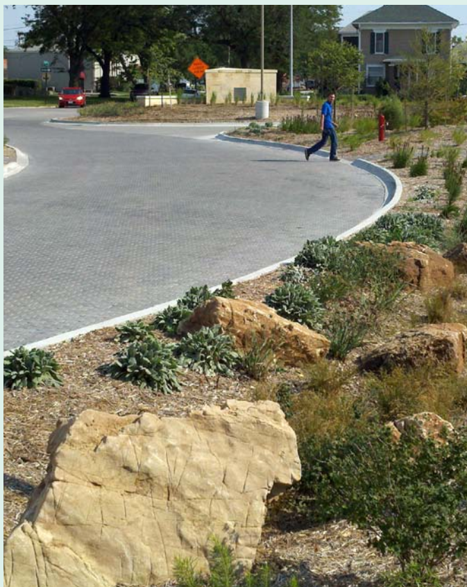
A SYSTEM OF NATIVE VEGETATION USED TO HELP ABSORB WATER AND CLEANSE IT AS IT IS SLOWED DOWN AND MOVES THROUGH THE SOIL PROFILE BEFORE REACHING A RIVER OR STREAM
